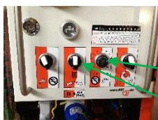
Pump motor switch / Speed switch
